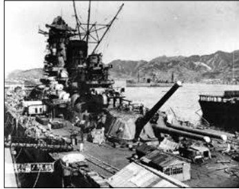
Battleship Yamato under construction (Source: Yamato Museum)
